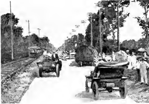
The first concrete paving was laid in Maryland in the summer of 1912. Here a hay wagon and a couple of flag-bedecked early cars try out the new surface.
